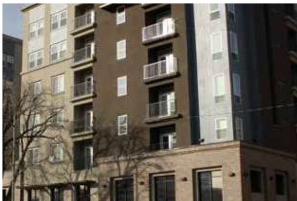
Figure 3.15 (5). Balconies Integral to Facade
