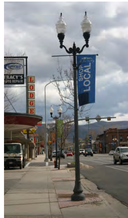
Fig 18: Existing Conditions: Lightpole & Luminaire
