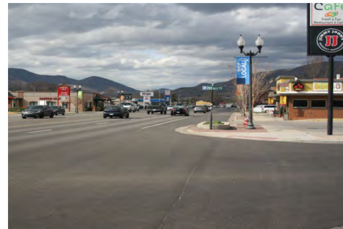
Fig 12: Existing Conditions - Missing Crosswalk Striping
