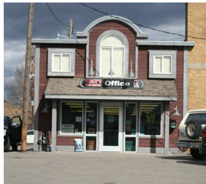
Fig 20: Existing Conditions - Main Street Façade Example
