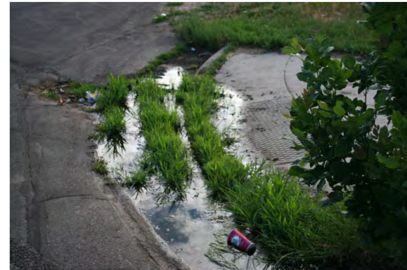
Fig 8: Existing ADA Ramp Within Project Area
