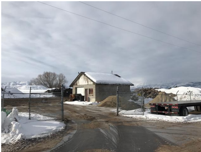
NORTH SIDE OF SUBJECT FACING SOUTH
