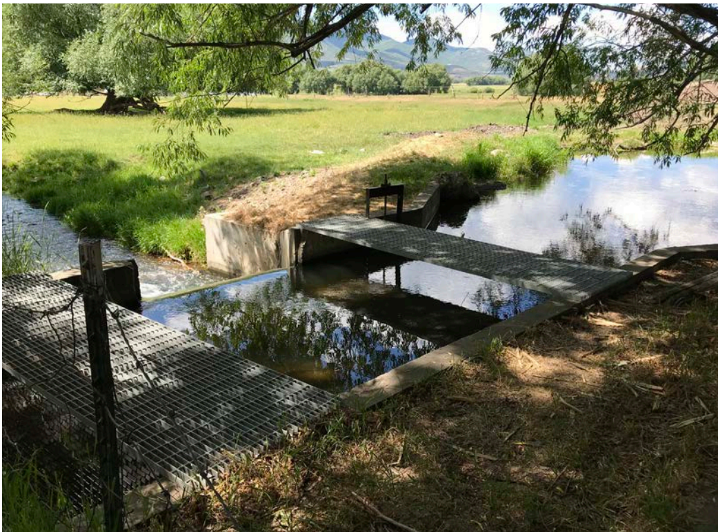
Photo 4. Site 42WA238, Sagebrush and Spring Creek Canal, modern diversion structure; view to the northwest.
